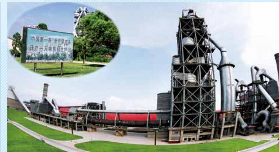
Conch Zongyang Cement Co., Ltd Phase 3 Line 1, China's first 10,000 t/d new dry process cement production line, operated in 2004
