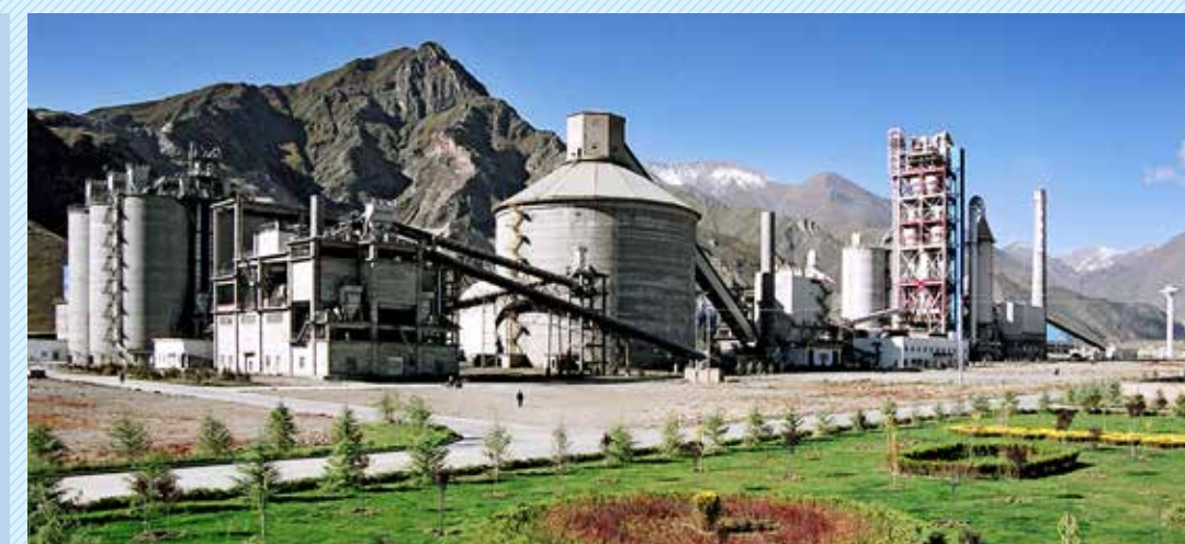
Tibet Gaozheng Building material Co., Ltd. 2,000t/d Project, the highest altitude new dry process cement production line in the world (elevation is 3720 meters) , operated in 2004
